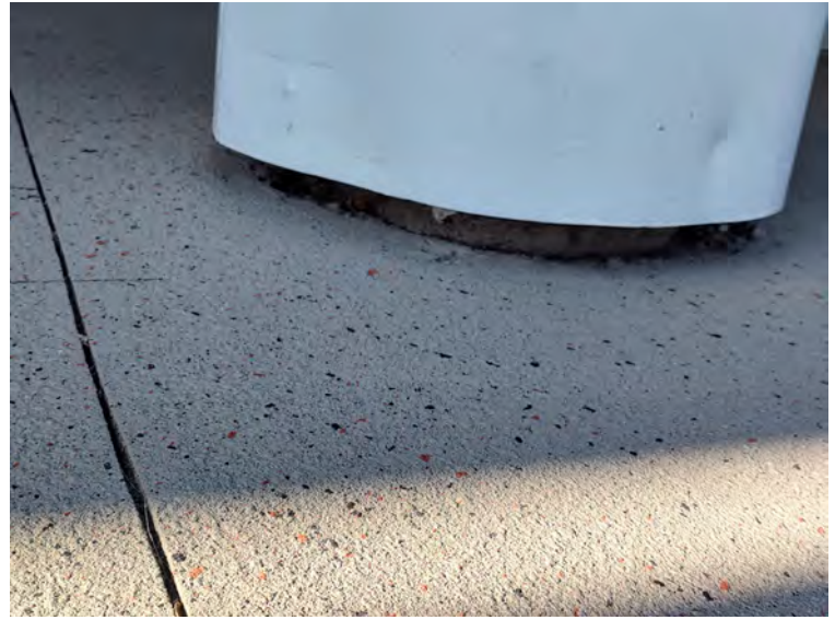
Bottom of concrete pillar
