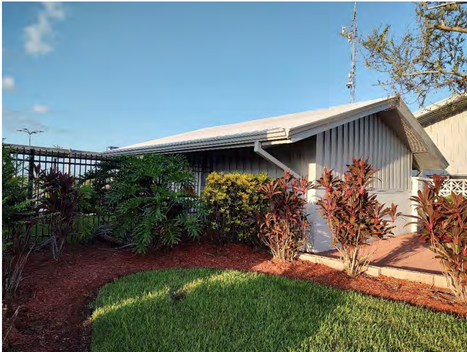
Figure 23 View southwest to Building M6-0409F
