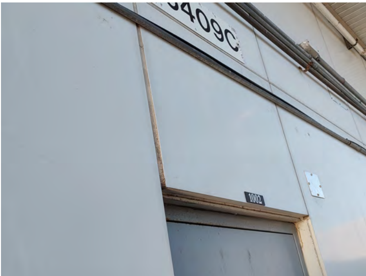
wall detail shot
