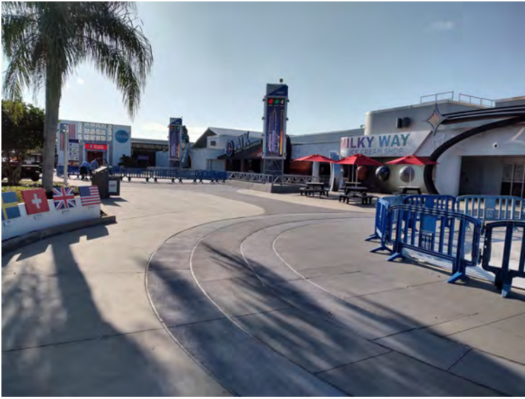
Overall north facade east end
