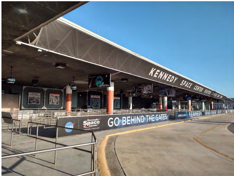
Figure 16 View northwest to east side of Bldg. M6-0409C
