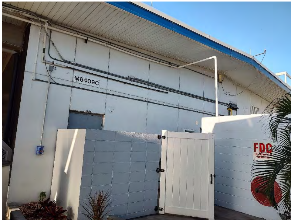
Figure 18 North side of Bldg. M6-409C
