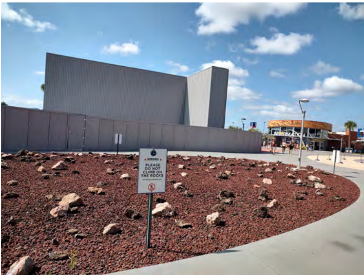
Facing south from south side_west end
