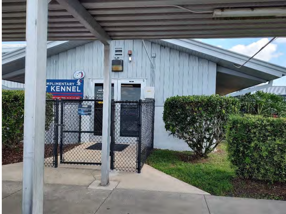
Figure 24 View north to Building M6-0409F
