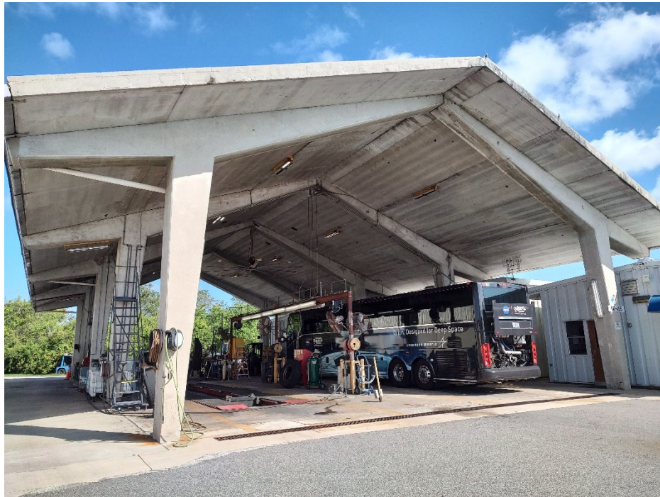
Figure 7. South Façade of M6-0455 Tour Bus Servicing
