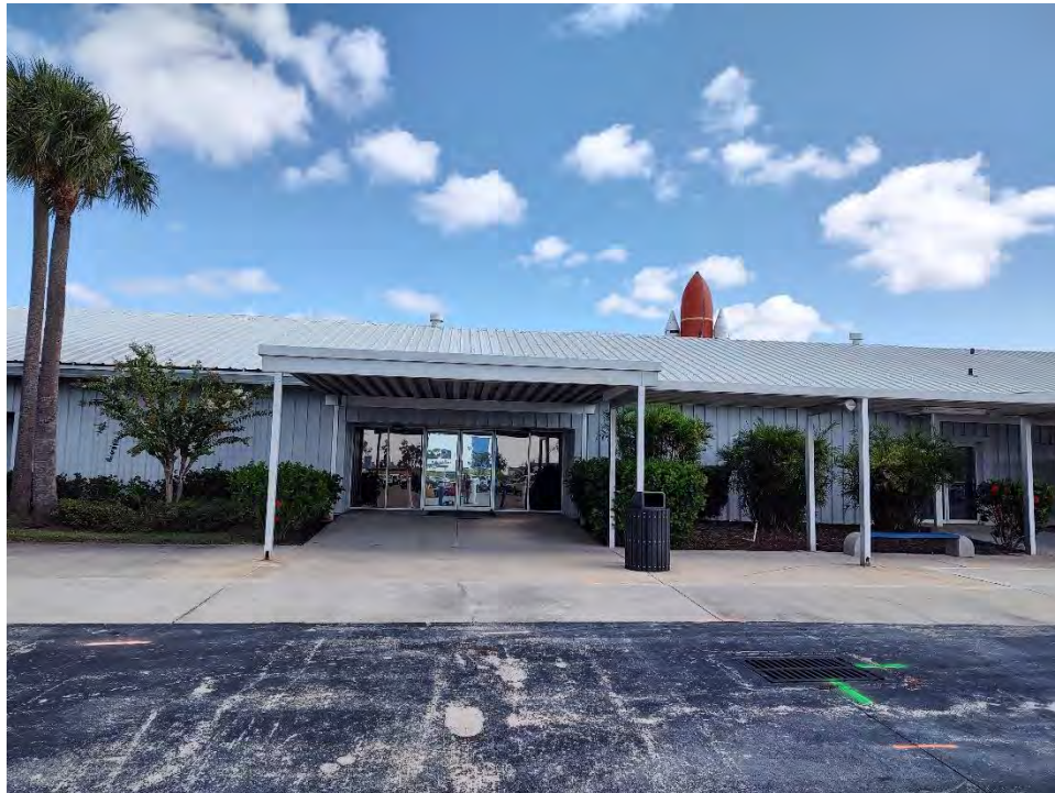
Figure 10 Bldg. M6-0409, view north to south facade, east addition
