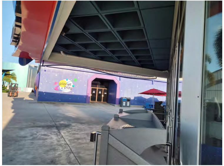
Facing west from northwest side
