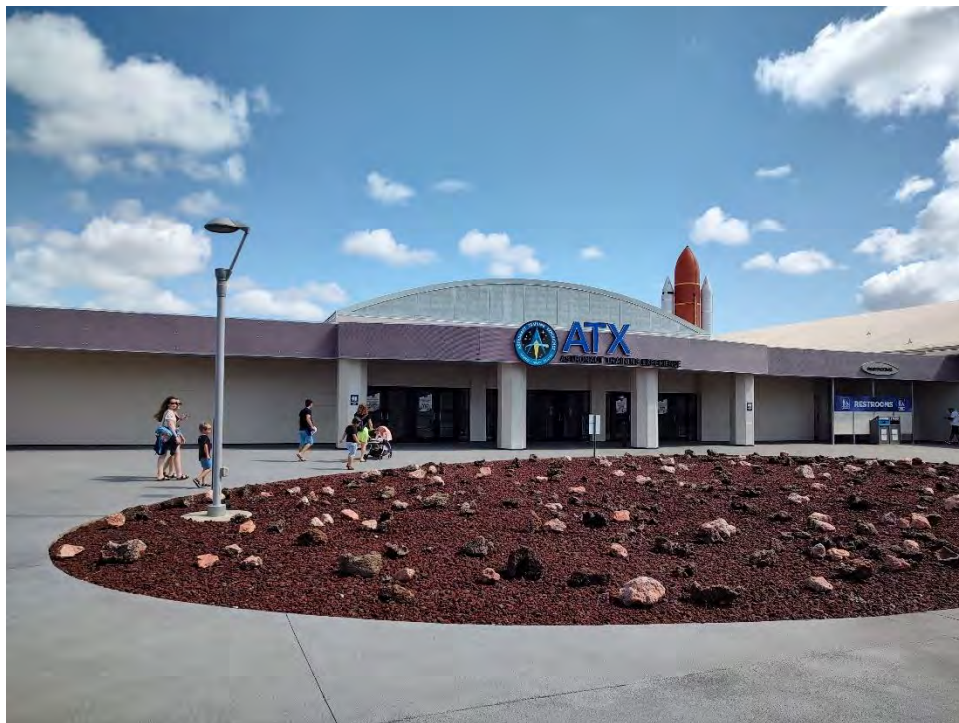
Figure 7 Bldg. M6-0409, view north to south façade, center bay (original main entrance)
