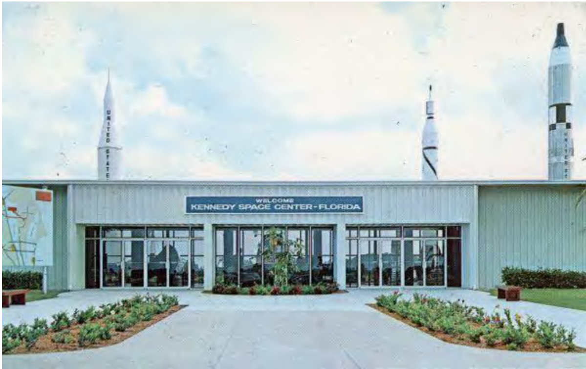
Figure 8 View of Bldg. M6-0409 entrance (Figure 11) in late 1960s (Florida Memory)
