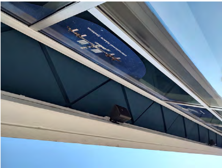
Detail shot of roof
