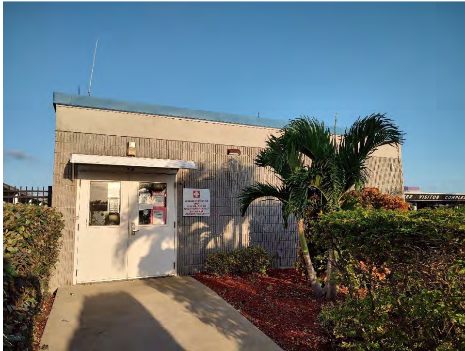
Figure 28 View west to Building M6-0411 facade
