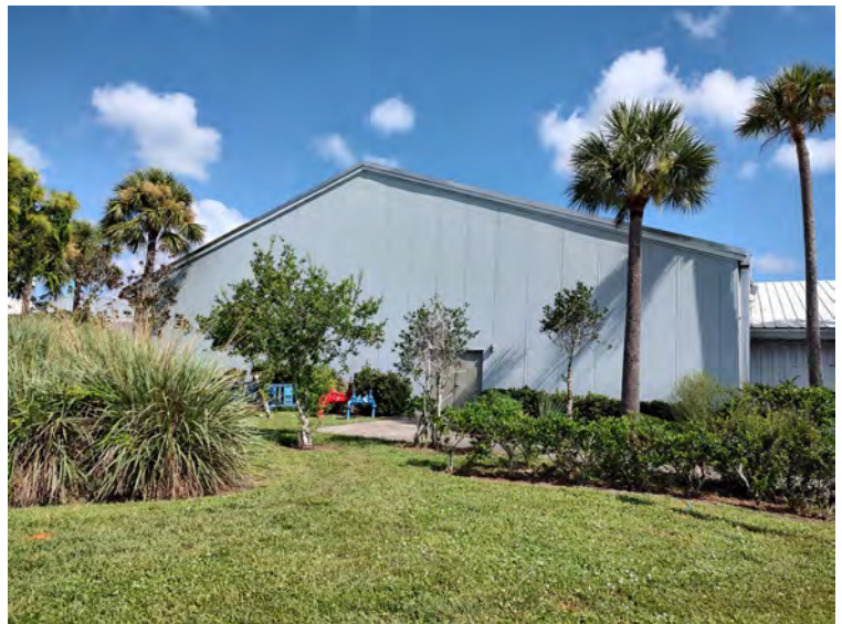
South facade east end
