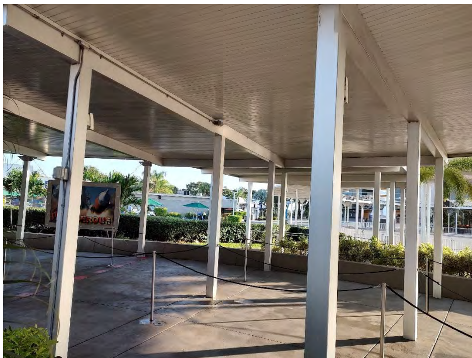
Figure 17 View north from north side of Bldg. M6-0409C showing wrap-around walkway
