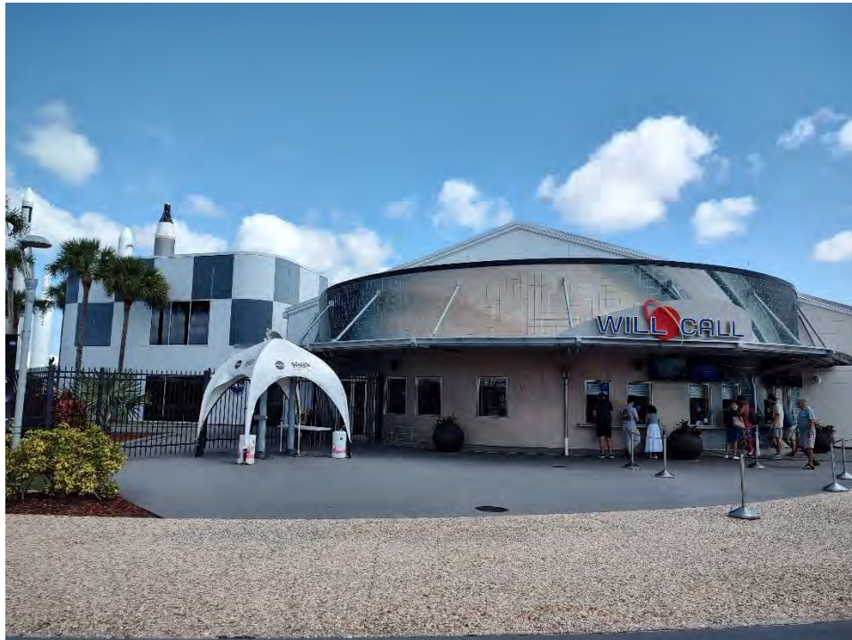
Figure 6 Bldg. M6-0409, view north to south façade, west end (note additions in foreground and left of photo)
