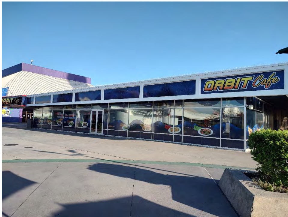
Figure 20 View northwest to Building M6-0409D
