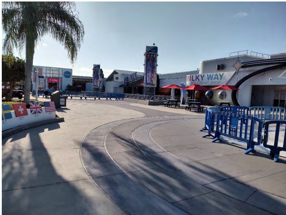
Figure 11 Bldg. M6-0409, view southeast to heavily modified south façade
