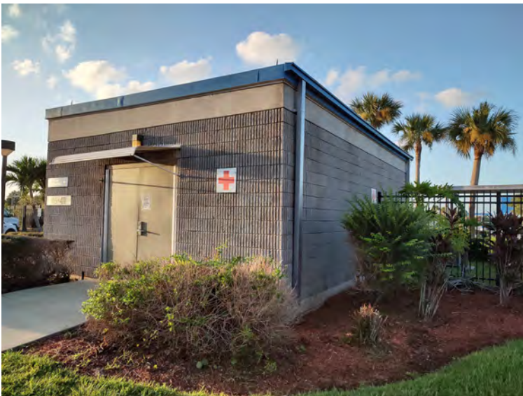
West and North facade
