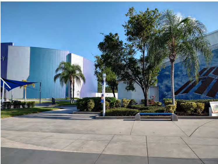
Facing north from north side_west end
