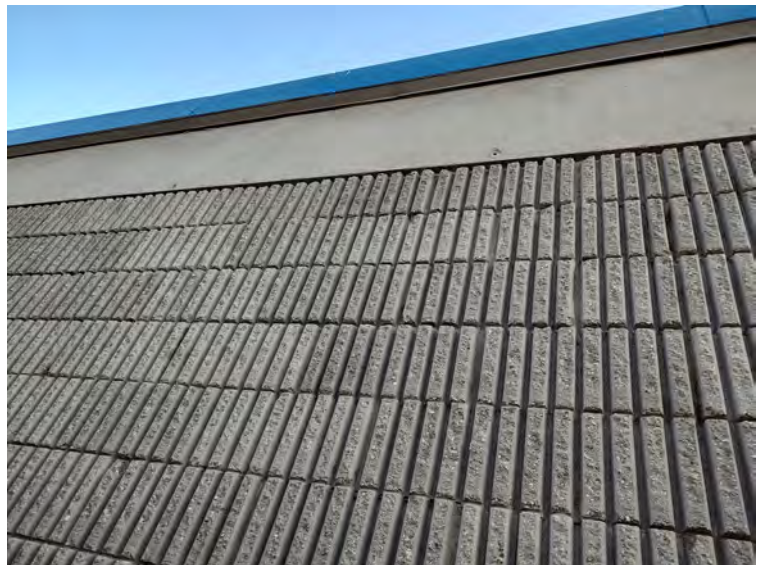
Detail shot of roof and wall
