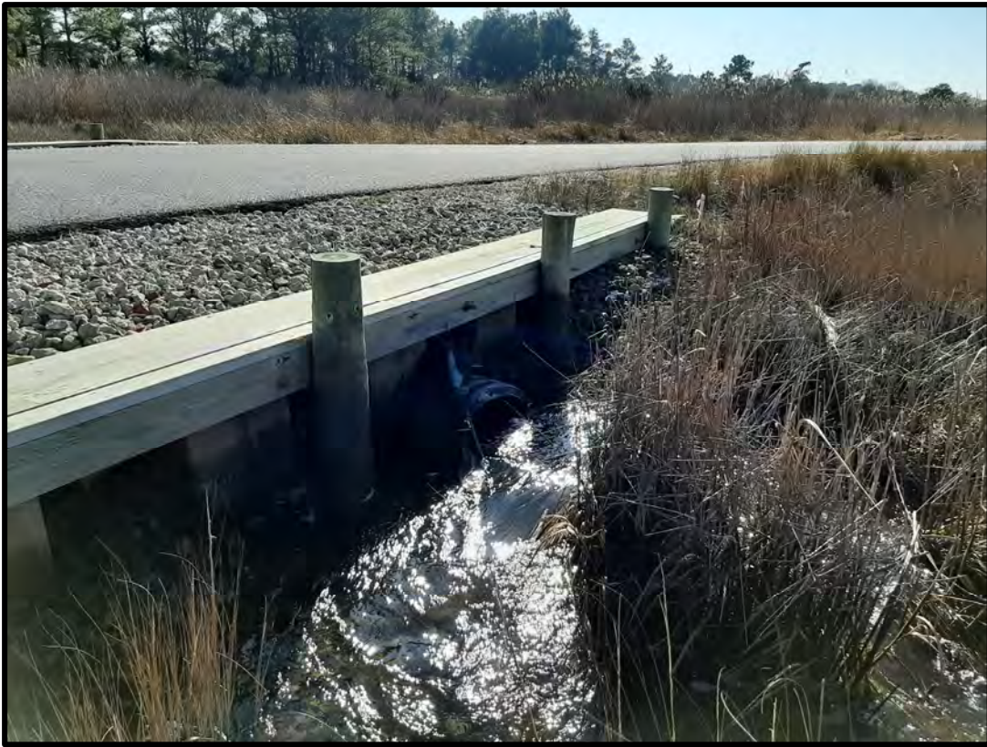
Photograph 9: Western side of culverted stream crossing
