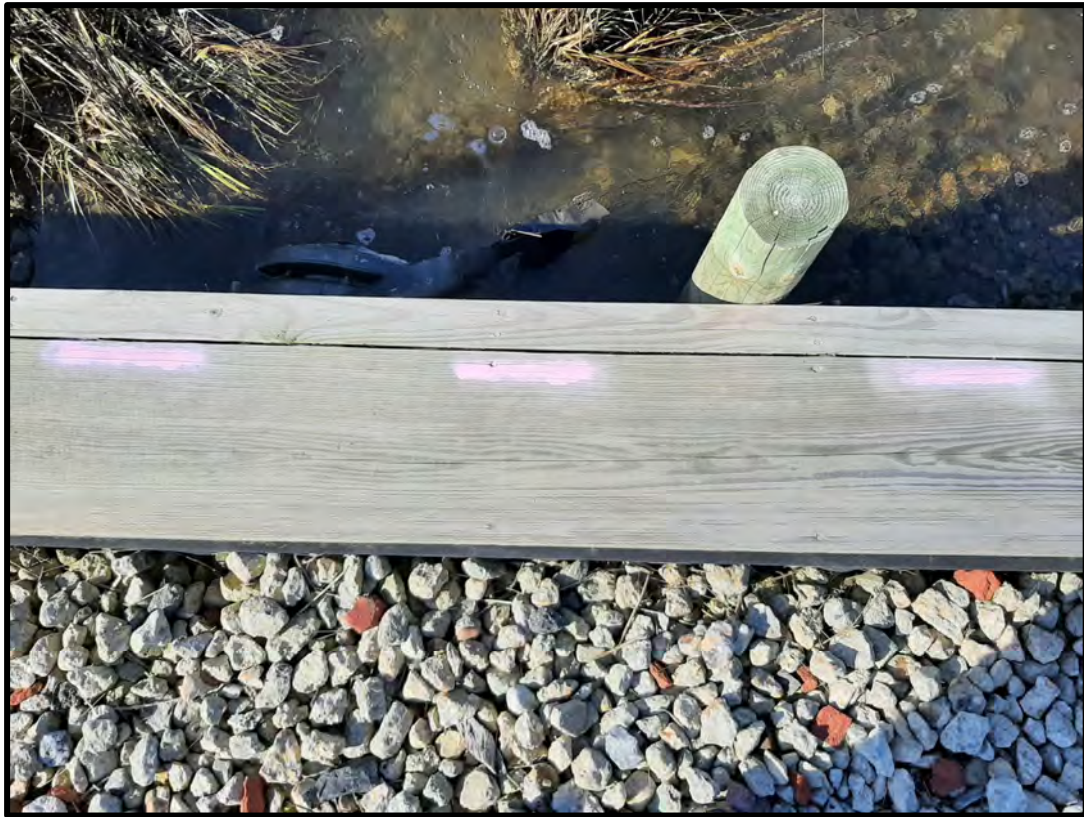
Photograph 7: Typical view of wetland line located directly above retaining wall
