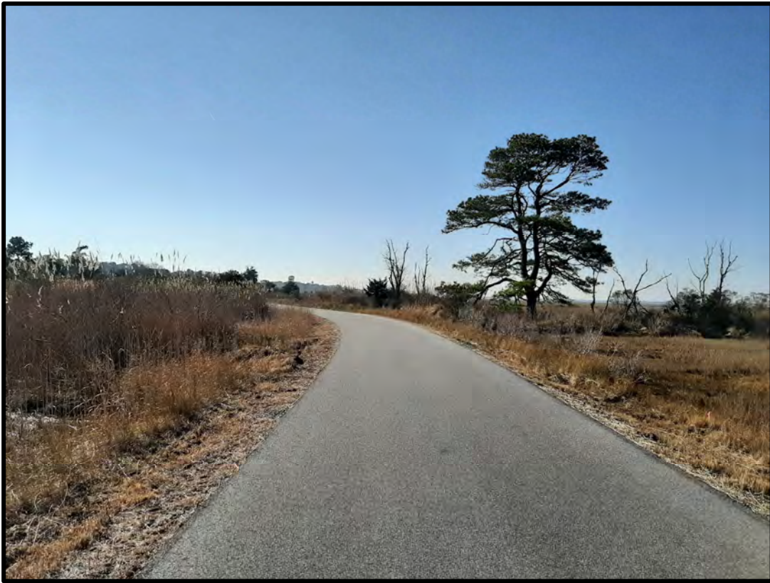
Photograph 5: Representative view of the roadway within the study area
