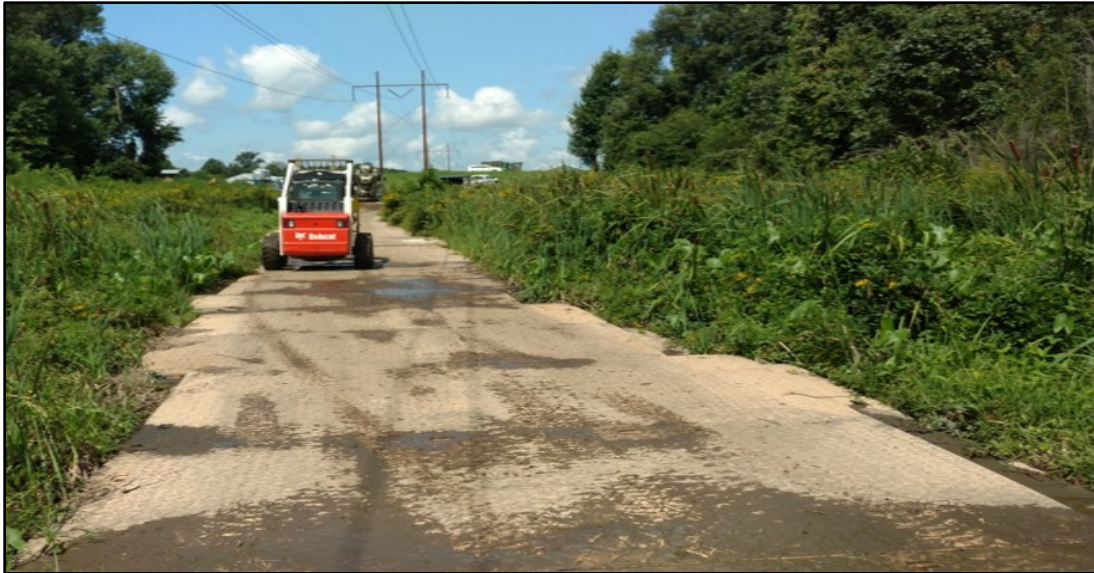
Photo 2-5. Example of matting to be used on Walker Marsh.
