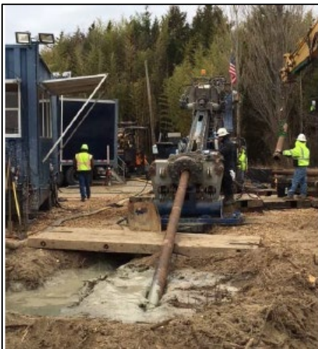
Photo 2-1. Example of Maxi HDD equipment drilling a borehole. Credit: Crofton Diving
