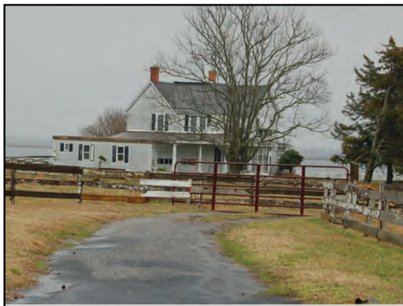
Photo 9. 33241 Taylor Farm Road does not retain integrity because of side addition, porch enclosures, and aluminum siding.
