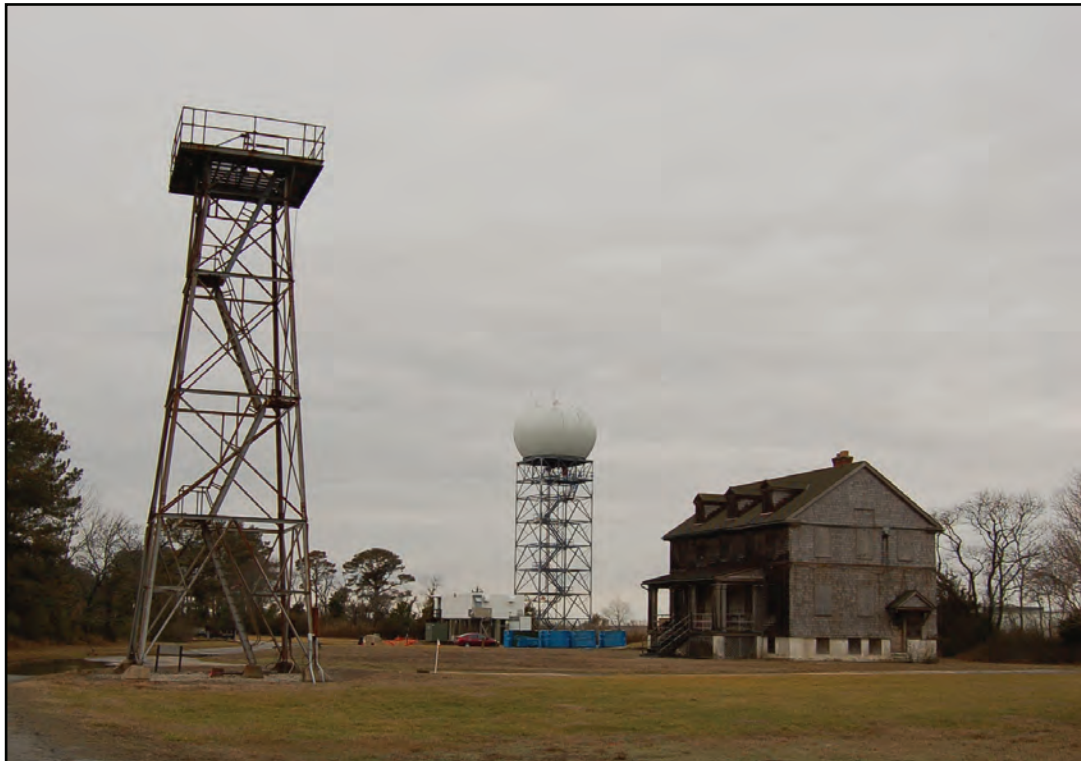
Photo 2. Wallops Beach Life Saving Station and Observation Tower, Looking Southwest
