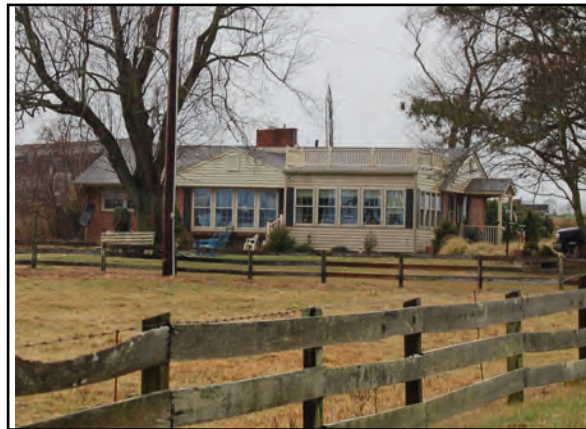
Photo 11. 33190 Taylor Farm Road does not retain integrity because of side addition, window replacement, and vinyl siding.
