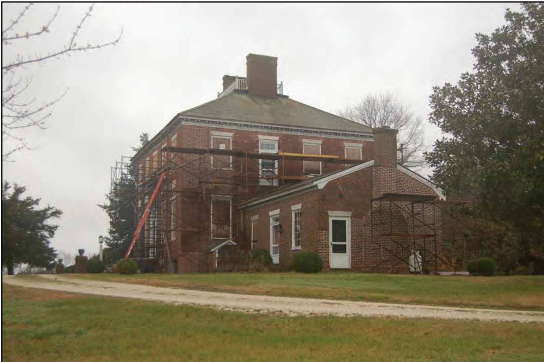
Photo 2. 13485 Wharton Drive, Looking Southwest
