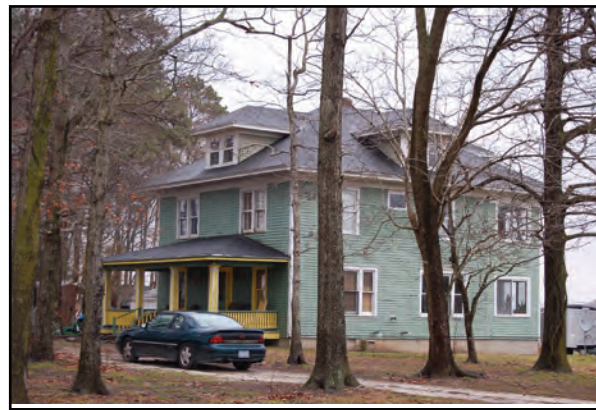
Photo 6. 32307 Mt. Wharton Road does not retain integrity because of window replacement, concrete block cladding at the foundation, and large two-story rear addition.
