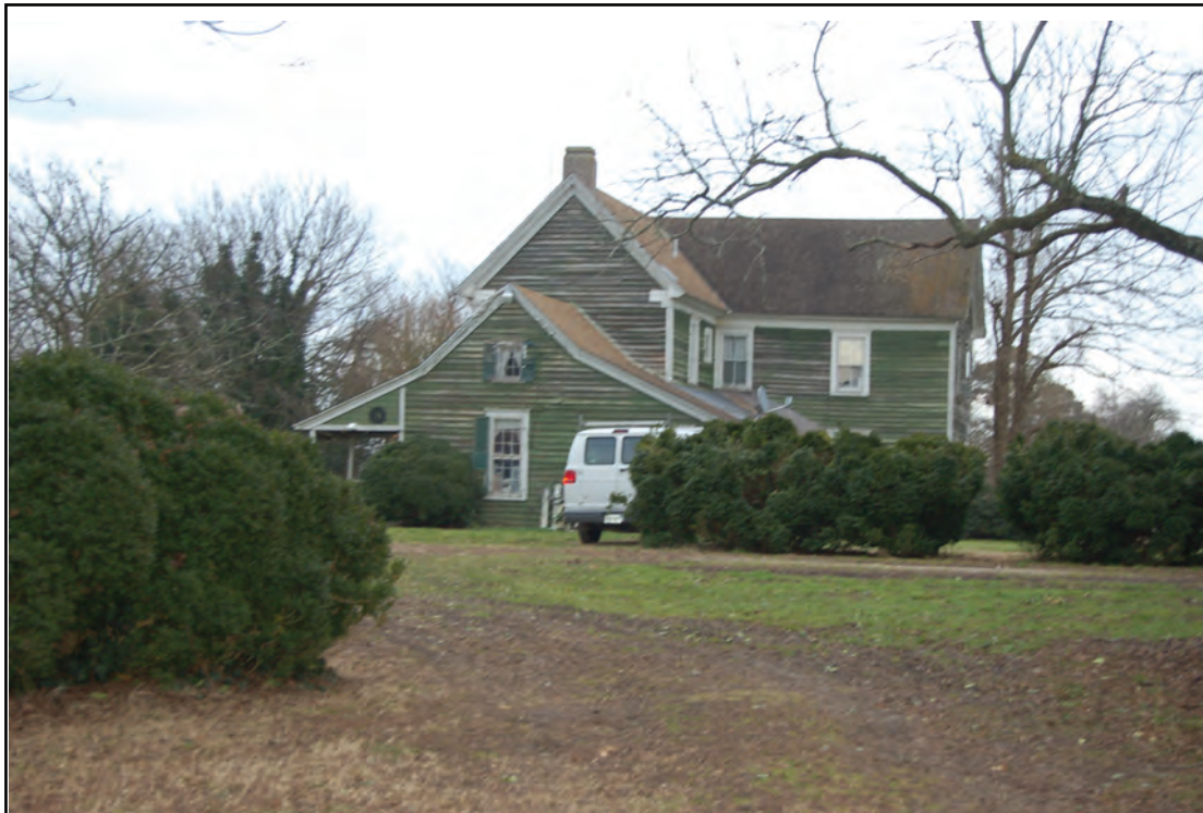
Photo 2. 31545 Point Breeze Lane, Looking Southeast
