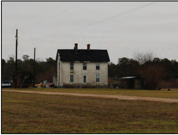
Photo 13. 32145 Wallops Island Road does not retain integrity because of asbestos siding, and rear porch enclosure.
