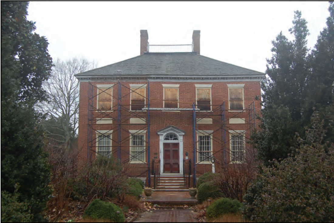
Photo 1. 13485 Wharton Drive, Looking Northwest
