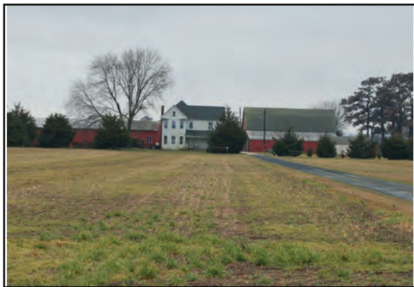
Photo 1. 13454 Arbuckle Neck Road does not retain integrity because of window replacement, rear additions, and asbestos siding.
