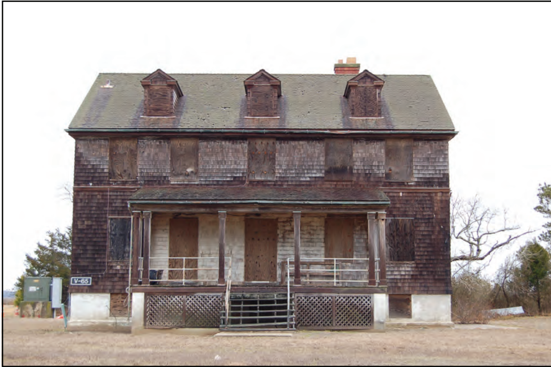
Photo 1. Wallops Beach Life Saving Station, Looking Northwest
