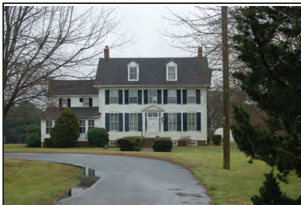
Photo 5. 13149 Metompkin Road does not retain integrity because of aluminum siding, porch enclosures, and large, two-story rear addition.
