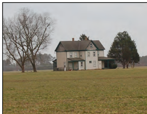
Photo 4. 31263 Mappsville Road does not retain integrity because of vinyl siding, window replacement, and porch enclosures.
