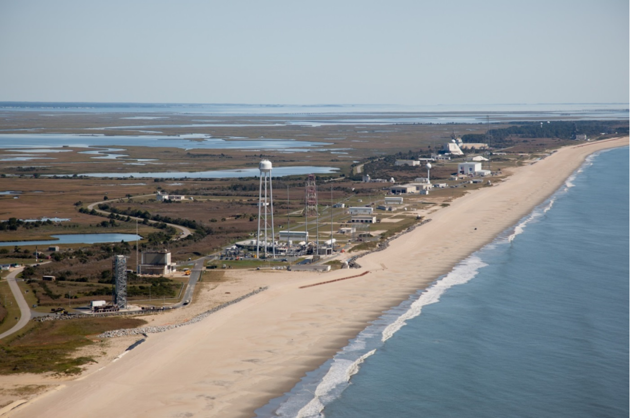
Figure 3-18: Variations in Structure Heights and Overall Visual Character of Wallops Island
