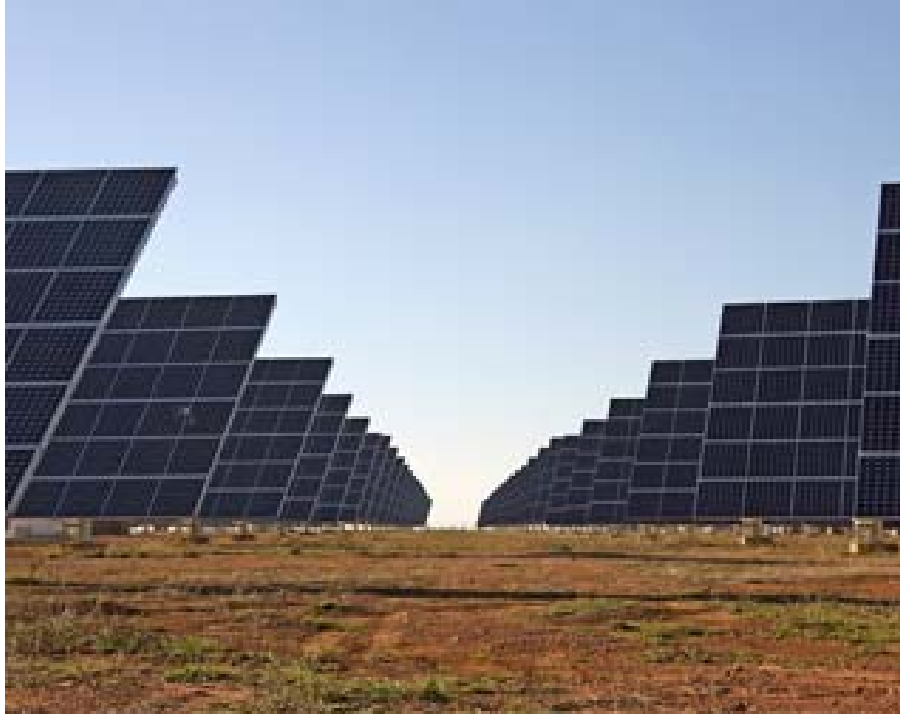
Figure 6 Tucson Electric Power Company Ground Array (4.6 MW on 44 acres [0.18 km 2 ])
