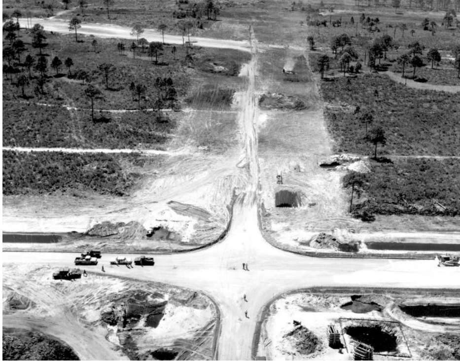
Figure 3.7 Construction Activity in the Industrial Area ca. 1965 (from Grinter 2007).
